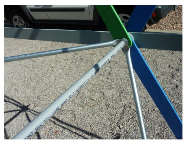
$^{3}\!\!/_{4}$  inch PVC was cut and sleeved over the  $^{1}\!\!/_{2}$  inch axles to prevent the bridge from collapsing in on itself. Some assembly required here.
