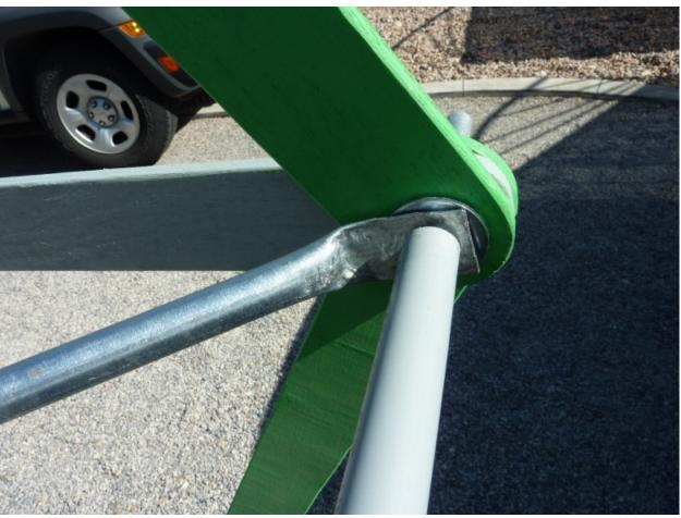
I used EMT compression pipe couplings cut in half to use as my axle locks. Only a pair of channel locks pliers and a crescent wrench are needed to tighten them.
